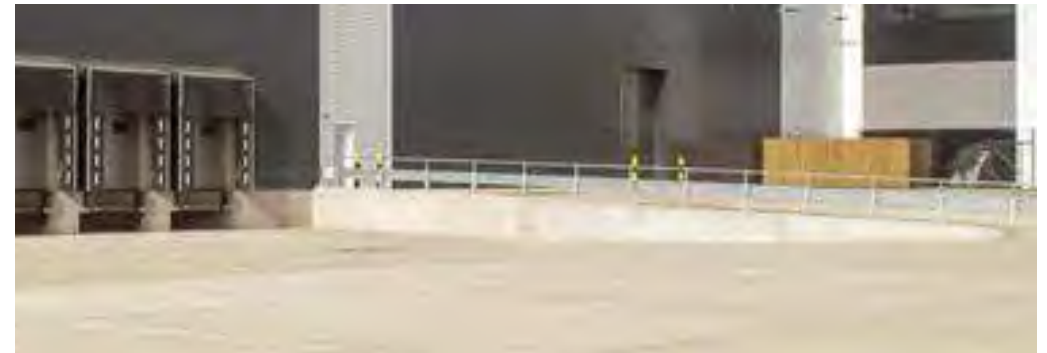
Precast concrete retaining walls to dock loading areas
