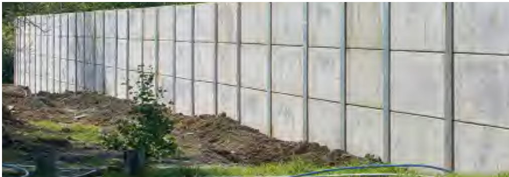
Kingpost retaining walls where walls arent visible from public areas
