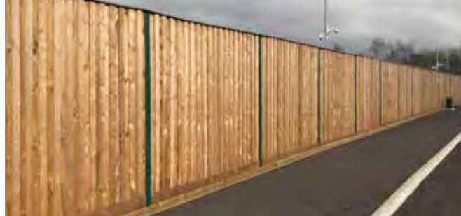
Typical Acoustic Fence
