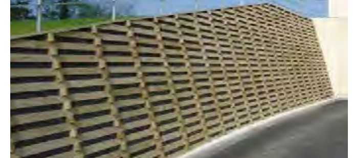
Cribblock retaining wall
